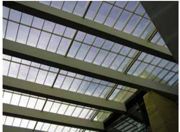
Glass ceiling with top-mounted track for regular cleaning and maintenance
