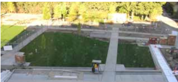
Natural-looking drainage feature for storm water collection and distribution
